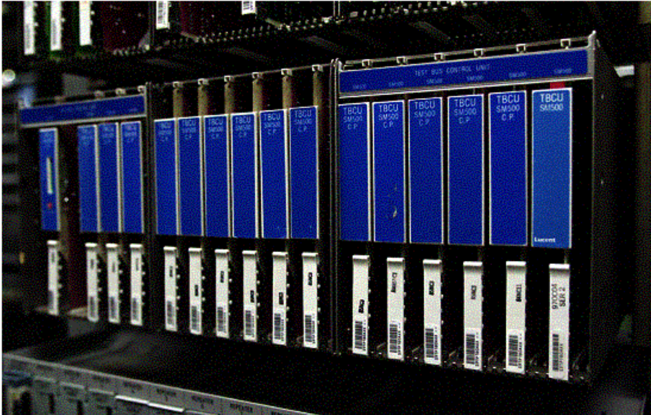
Figure 5•3 Test Bus Control Unit (TBCU) Shelf
