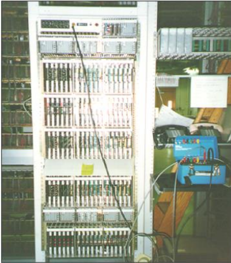
Figure 2•2 Fully Installed LTS Rack
